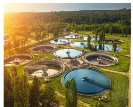
Sewage & Water Treatment Plants
