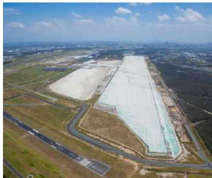
Airports & Railway Station Slab Reinforcement
