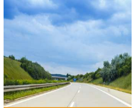
Highways & RCC Road Slab Reinforcement
