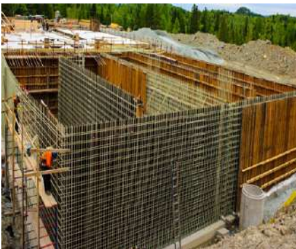
STP Structure Reinforcement
